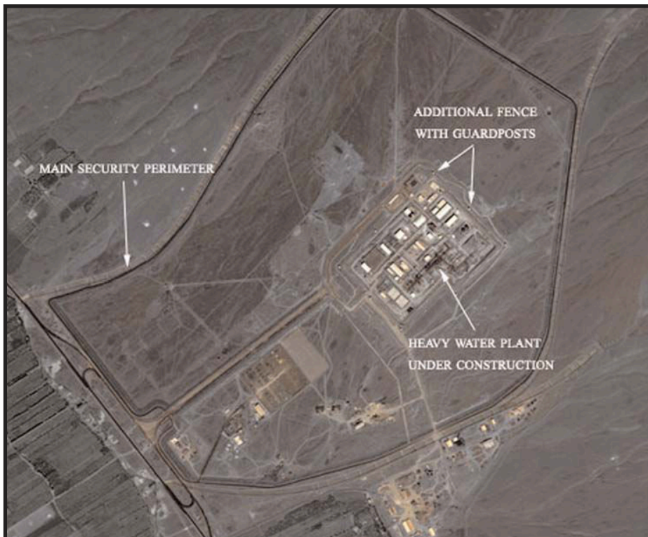
The Arak site is a potential heavy water production facility, and is located about 150 miles south of Tehran.
